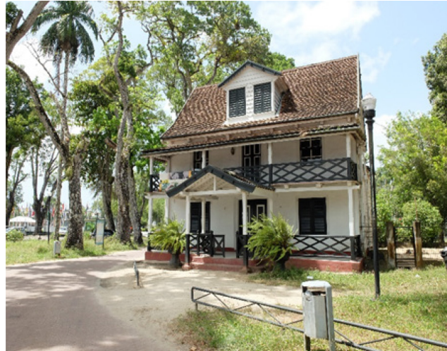
Abb. 5: Kolonialhaus am Fort Zeelandia (LEBMAN 2019)
