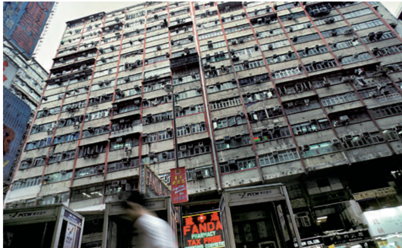
2 Chungking Mansion in Kowloon/Hongkong (China); Foto: Nils Mevenkamp
